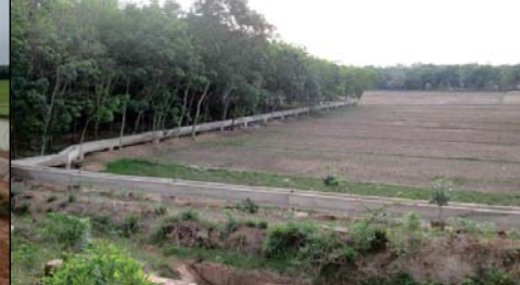
三次水路 Aqueduct Flume Type L=23.7 km
