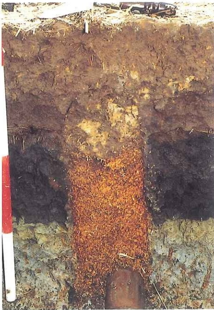
Underdrain in paddy field (rice husks as surround material of a drain pipe)
