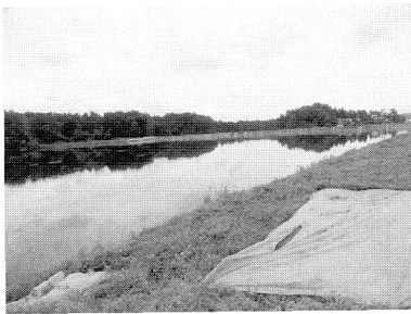
(a) 堤体の亀裂 (大池, 刈羽村井岡)
